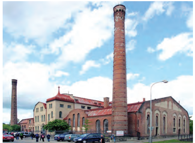
The impressive building at Bubeneč, showing the twin chimneys. One was a conventional boiler smokestack, the other was used to exhaust foul air
